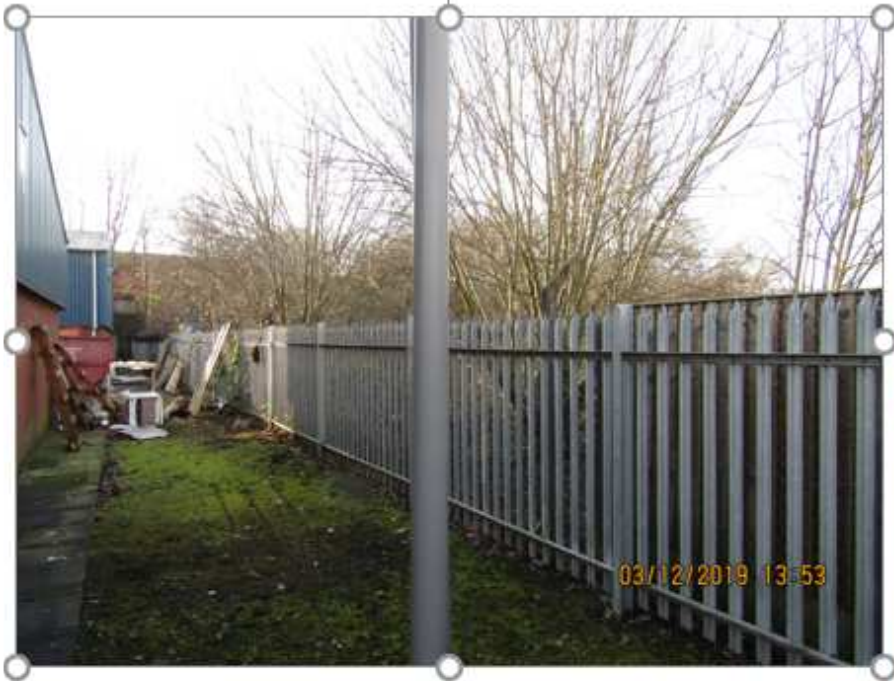
South-eastern edge of site
